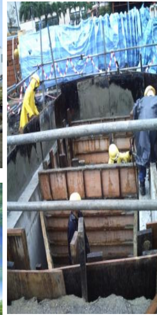
Sept 2010: Commencement of piling works
