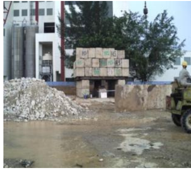
Aug 2010: Completion of demolition works
