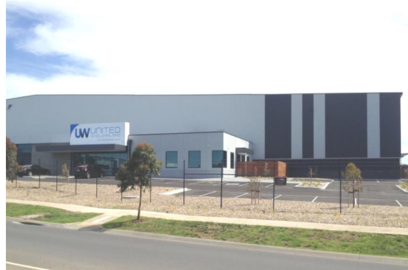
169-177 Australis Drive, Derrimut, Melbourne
