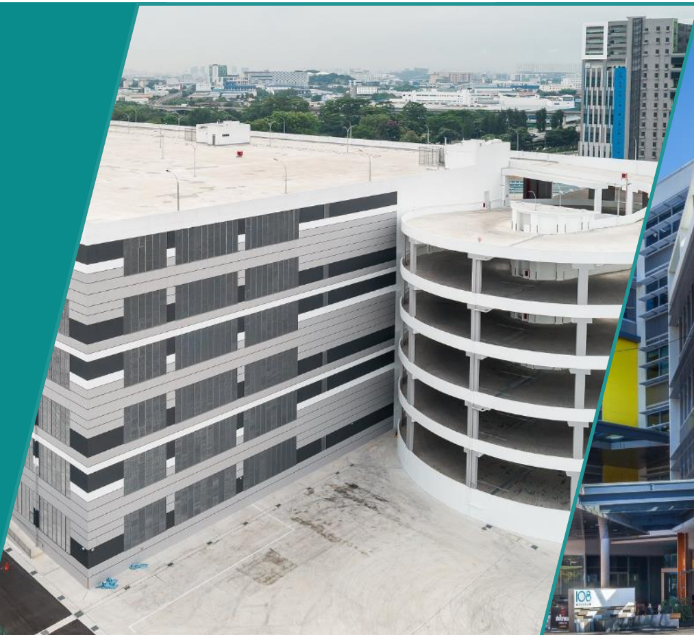
20 Tuas Avenue 1 Singapore
