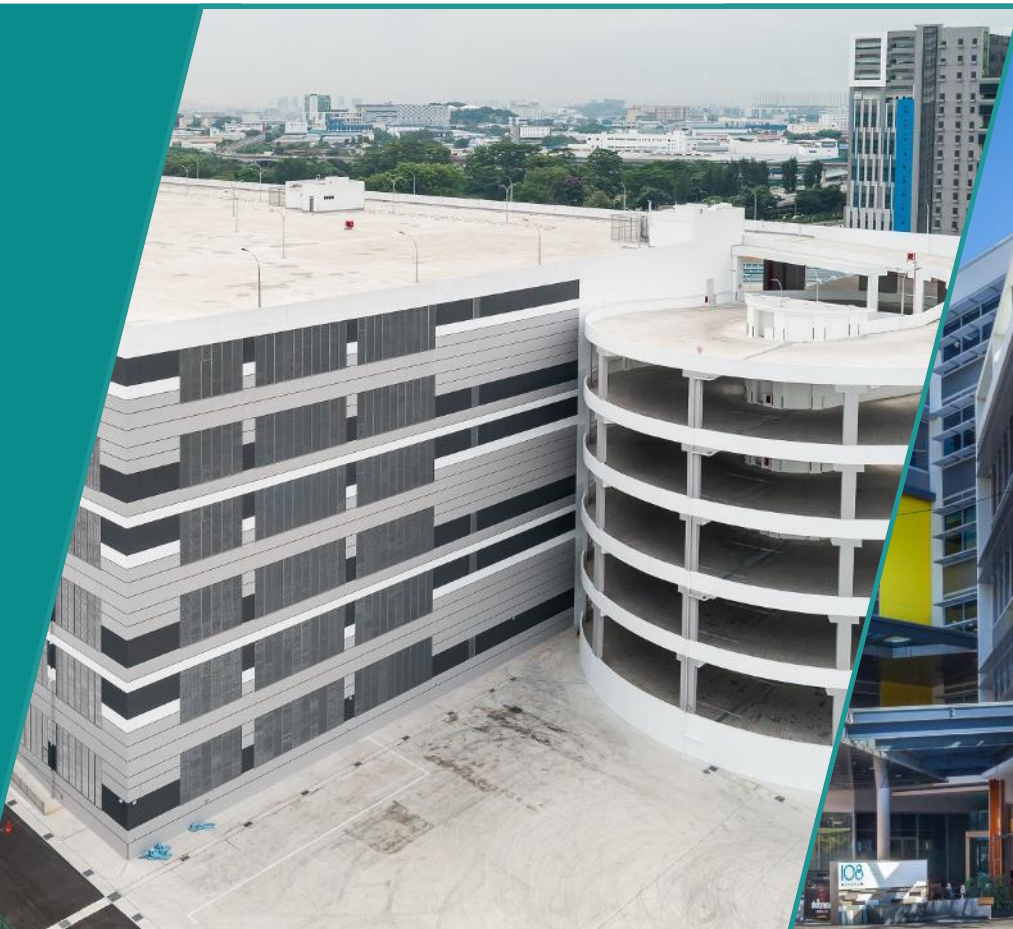
20 Tuas Avenue 1 Singapore
