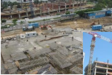
Sept 08: Commenced construction of MTB Building
