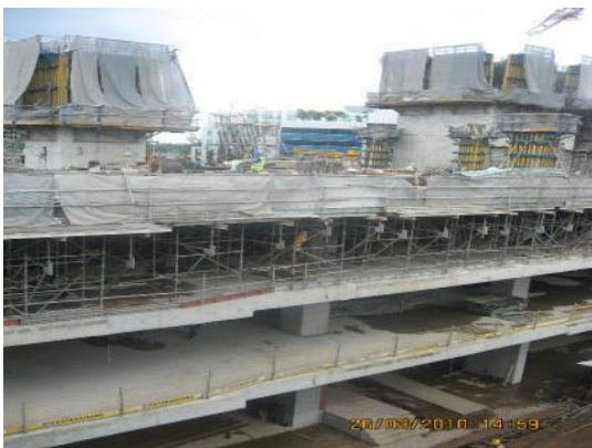
Phase2 Plot 8 Changi Business Park at 3 Changi Business Park under construction
