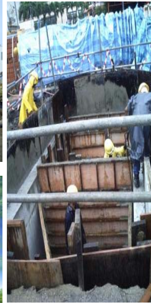
Sept 2010: Commencement of piling works
