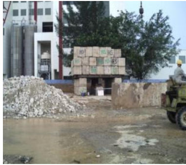
Aug 2010: Completion of demolition works
