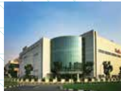
93. Xilin Districentre Building D
