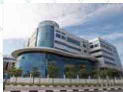
49. 2 Changi South Lane
