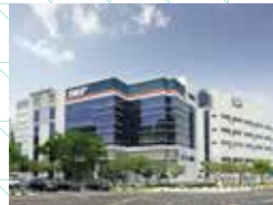
98. 1 Changi South Lane
