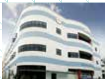
72. NNB Industrial Building
