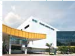
88. Changi Logistics Centre
