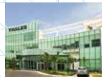
75. Thales Building (I & II)
