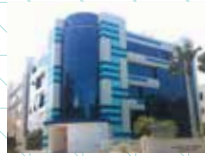
56. 41 Changi South Avenue 2
