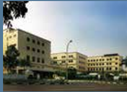
87. Xilin Districentre Building A&B
