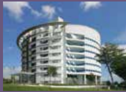
31. Kim Chuan Telecommunications Complex
