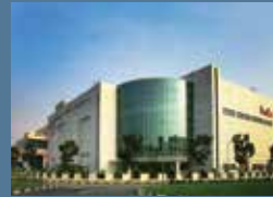
89. Xilin Districentre Building D
