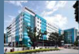
90. 9 Changi South Street 3
