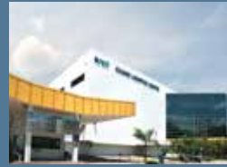
84. Changi Logistics Centre
