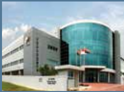
96. Serial I-Tech Building (formerly GSH Centre)
