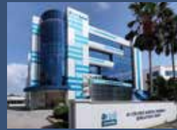
54. 41 Changi South Avenue 2
