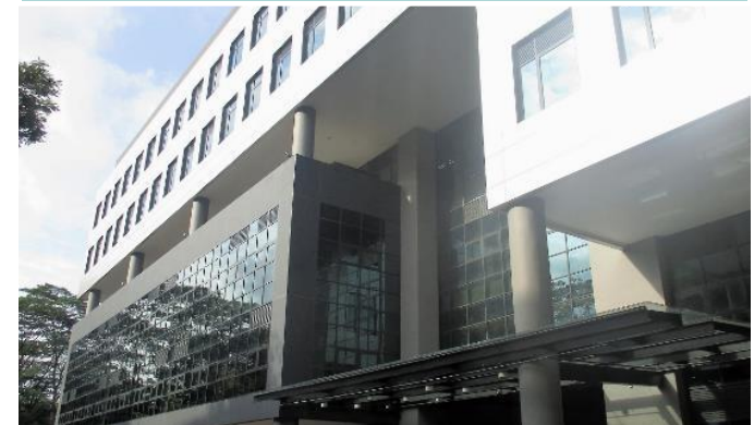
Painting & façade cladding
