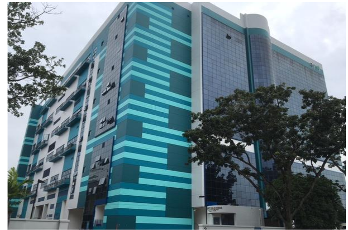
Completed façade painting
