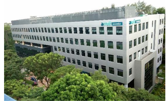
Completed façade cladding
