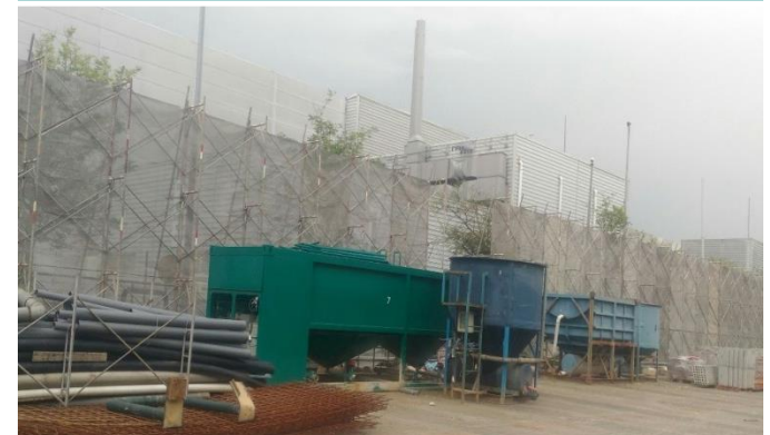
On-going works at site
