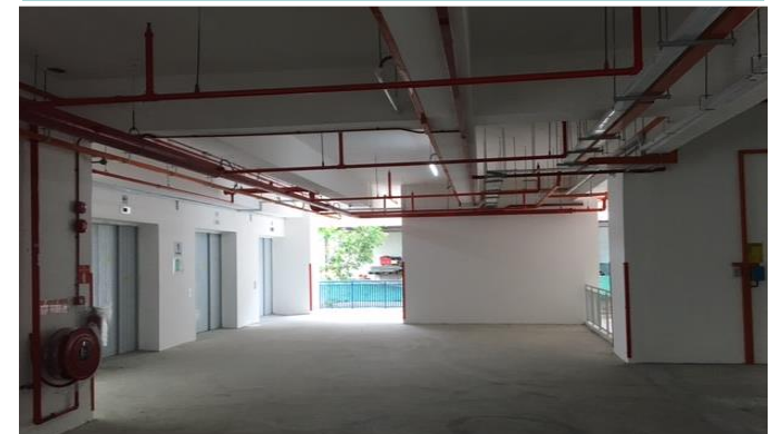
New cargo lift lobby
