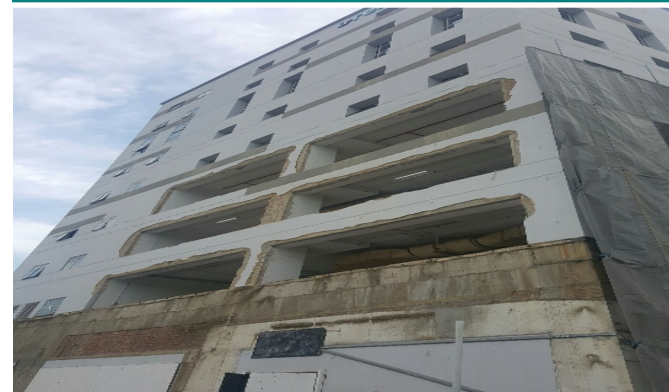
On-going works at site
