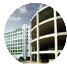
93. 19 & 21 Pandan Avenue (formerly Senkee Logistics Hub (Phase I & II))
