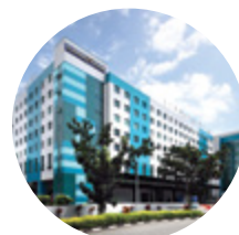
90. 9 Changi South Street 3
