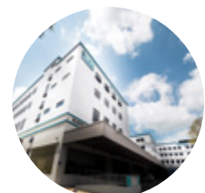
87. Xilin Districentre Building A&B
