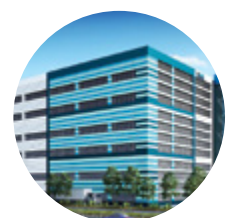
81. 20 Tuas Avenue 1 (formerly IDS Logistics Corporate HQ)
