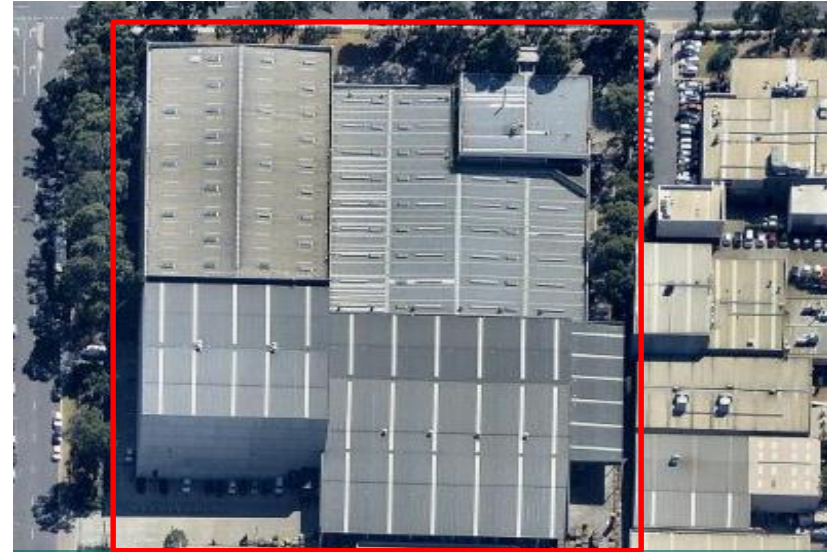
1314 Ferntree Gully Drive, Melbourne
