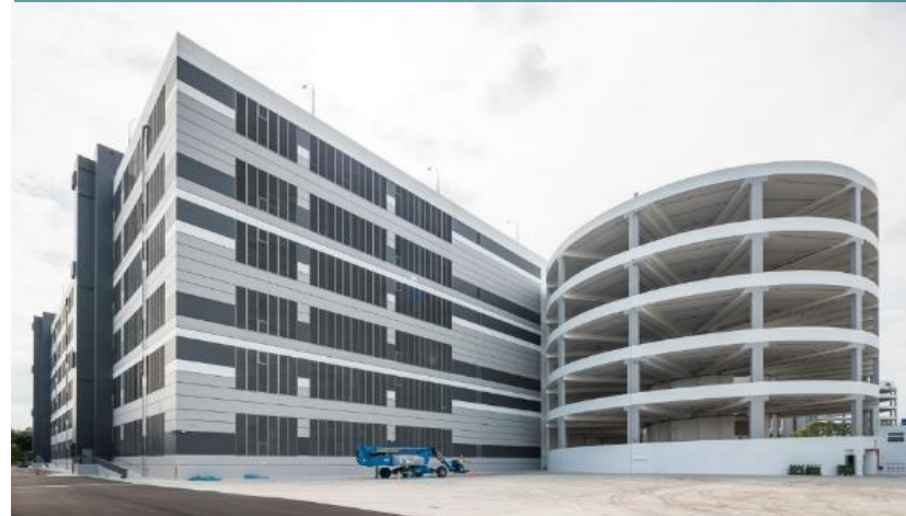
Warehouse Block and Ramp
