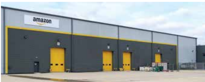
▲ Units 1a, 1b, 2 & 3 Upwell Street, United Kingdom
