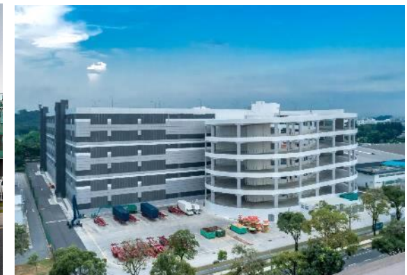
20 Tuas Avenue 1, Singapore
