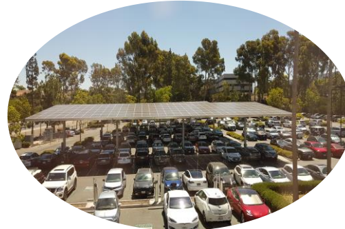
Solar panels used as carpark shelter
