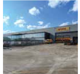
142 Units 1 - 2, Tower Lane
