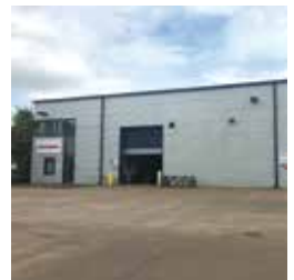
162 Unit 17, Wellesbourne Distribution Park
