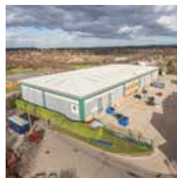
166 Unit 21, Wellesbourne Distribution Park
