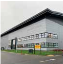
153 Unit 1, Wellesbourne Distribution Park
