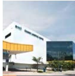
78 Changi Logistics Centre
