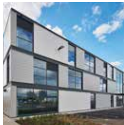
154 Unit 2, Wellesbourne Distribution Park
