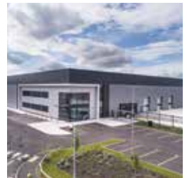
157 Unit 5, Wellesbourne Distribution Park
