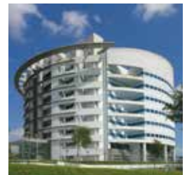
50 Kim Chuan Telecommunications Complex
