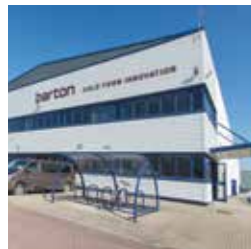
151 Unit 402, Stonebridge Cross Business Park
