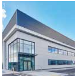
156 Unit 4, Wellesbourne Distribution Park
