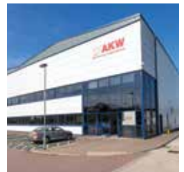
152 Unit 404, Stonebridge Cross Business Park
