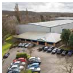
165 Unit 20, Wellesbourne Distribution Park
