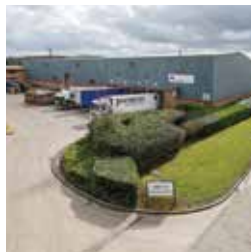
159 Unit 13, Wellesbourne Distribution Park
