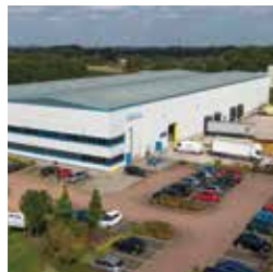
150 Unit 401, Stonebridge Cross Business Park
