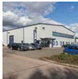
161 Unit 16, Wellesbourne Distribution Park
