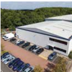
148 Unit 103, Stonebridge Cross Business Park
