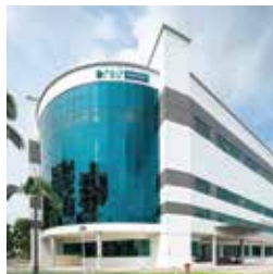
92 21 Changi South Avenue 2
