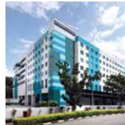
84 9 Changi South Street 3
