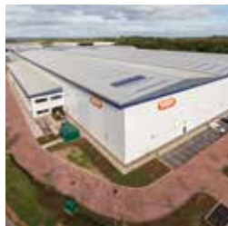
149 Unit 302, Stonebridge Cross Business Park
