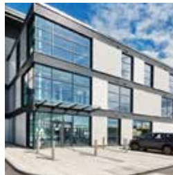
155 Unit 3, Wellesbourne Distribution Park
