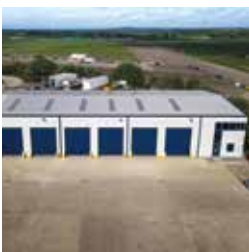
163 Unit 18, Wellesbourne Distribution Park
