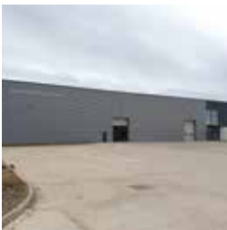
158 Unit 8, Wellesbourne Distribution Park
