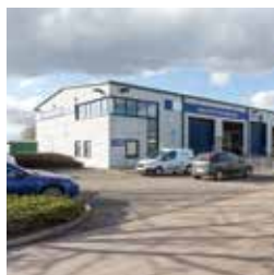
164 Unit 19, Wellesbourne Distribution Park
