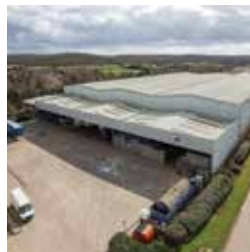
160 Unit 14, Wellesbourne Distribution Park
