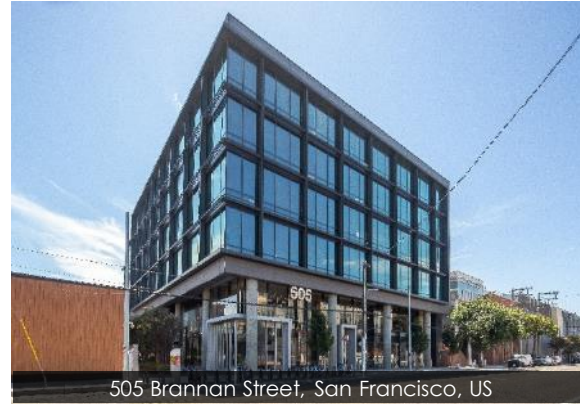
505 Brannan Street, San Francisco, US
