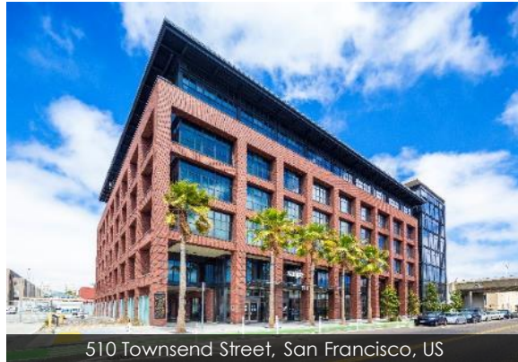
510 Townsend Street, San Francisco, US
