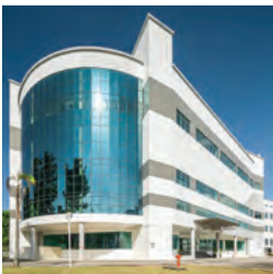
92 21 Changi South Avenue 2
