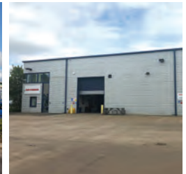
171 Unit 17, Wellesbourne Distribution Park
