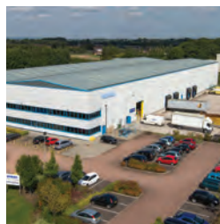
159 Unit 401, Stonebridge Cross Business Park
