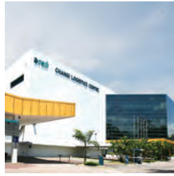
79 Changi Logistics Centre
