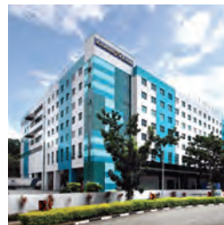
85 9 Changi South Street 3
