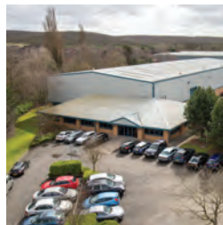
174 Unit 20, Wellesbourne Distribution Park
