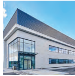
165 Unit 4, Wellesbourne Distribution Park
