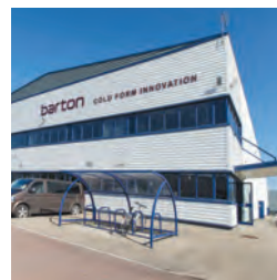
160 Unit 402, Stonebridge Cross Business Park
