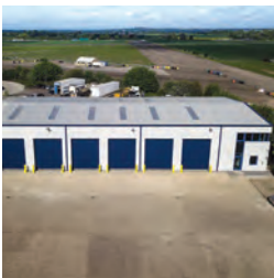
172 Unit 18, Wellesbourne Distribution Park
