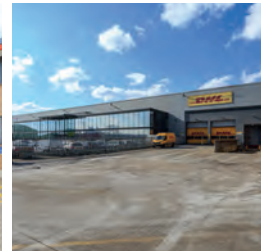
151 Units 1-2, Tower Lane
