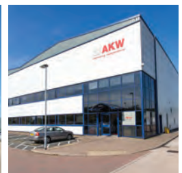
161 Unit 404, Stonebridge Cross Business Park
