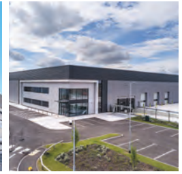
166 Unit 5, Wellesbourne Distribution Park
