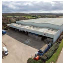
169 Unit 14, Wellesbourne Distribution Park
