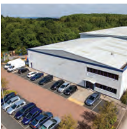
157 Unit 103, Stonebridge Cross Business Park
