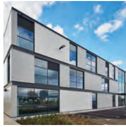
163 Unit 2, Wellesbourne Distribution Park
