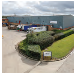
168 Unit 13, Wellesbourne Distribution Park
