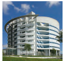
51 Kim Chuan Telecommunications Complex
