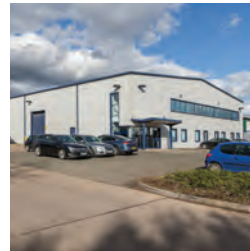
170 Unit 16, Wellesbourne Distribution Park
