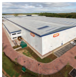
158 Unit 302, Stonebridge Cross Business Park
