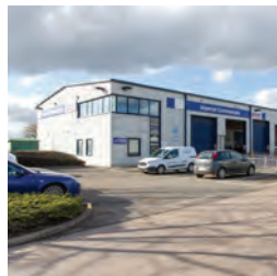
173 Unit 19, Wellesbourne Distribution Park
