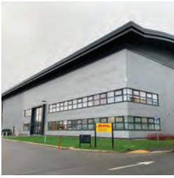
162 Unit 1, Wellesbourne Distribution Park
