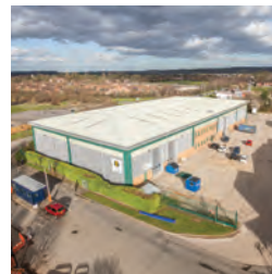
175 Unit 21, Wellesbourne Distribution Park
