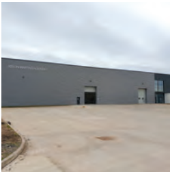
167 Unit 8, Wellesbourne Distribution Park
