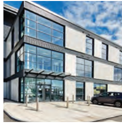
164 Unit 3, Wellesbourne Distribution Park
