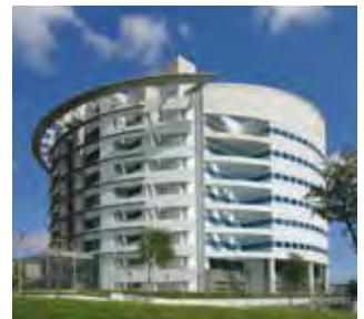
72 Kim Chuan Telecommunications Complex
