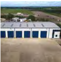
210 Unit 18, Wellesbourne Distribution Park
