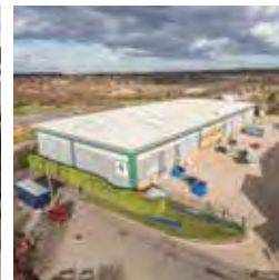
213 Unit 21, Wellesbourne Distribution Park
