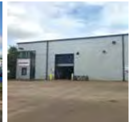
209 Unit 17, Wellesbourne Distribution Park
