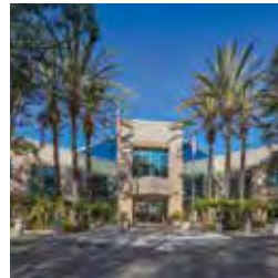
159 6055 Lusk Boulevard (decommissioned for major refurbishment work)
