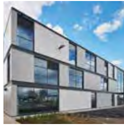
201 Unit 2, Wellesbourne Distribution Park
