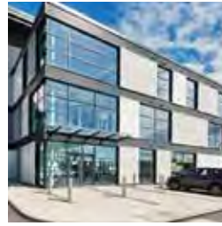
202 Unit 3, Wellesbourne Distribution Park
