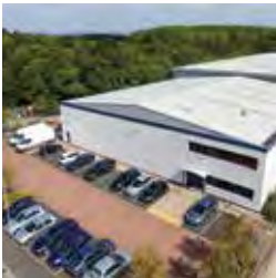
195 Unit 103, Stonebridge Cross Business Park
