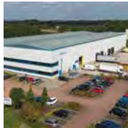
197 Unit 401, Stonebridge Cross Business Park
