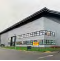
200 Unit 1, Wellesbourne Distribution Park
