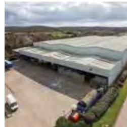
207 Unit 14, Wellesbourne Distribution Park
