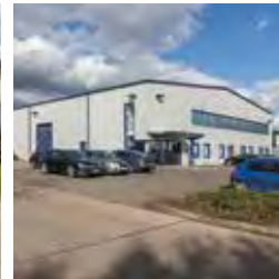
208 Unit 16, Wellesbourne Distribution Park
