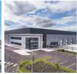
204 Unit 5, Wellesbourne Distribution Park
