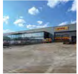
189 Units 1-2, Tower Lane
