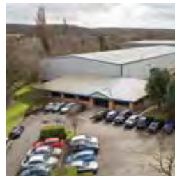
212 Unit 20, Wellesbourne Distribution Park
