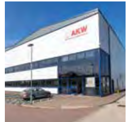
199 Unit 404, Stonebridge Cross Business Park
