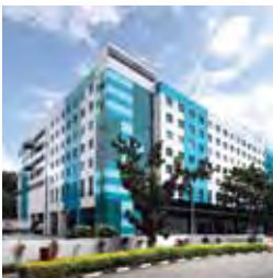
84 9 Changi South Street 3
