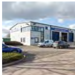
211 Unit 19, Wellesbourne Distribution Park
