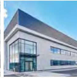
203 Unit 4, Wellesbourne Distribution Park
