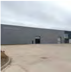
205 Unit 8, Wellesbourne Distribution Park
