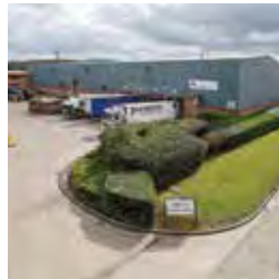
206 Unit 13, Wellesbourne Distribution Park
