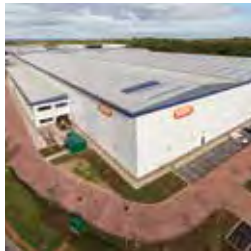
196 Unit 302, Stonebridge Cross Business Park
