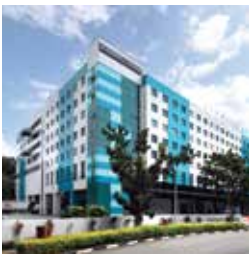
84 9 Changi South Street 3
