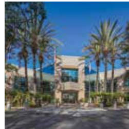
159 6055 Lusk Boulevard (decommissioned for major refurbishment work)
