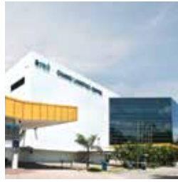
76 Changi Logistics Centre
