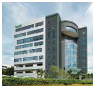
42 Schneider Electric Building
