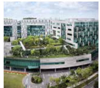
12 1, 3 & 5 Changi Business Park Crescent
