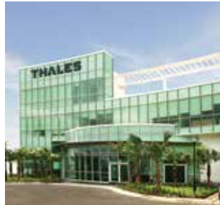
63 Thales Building ( I & II )
