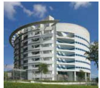
72 Kim Chuan Telecommunications Complex
