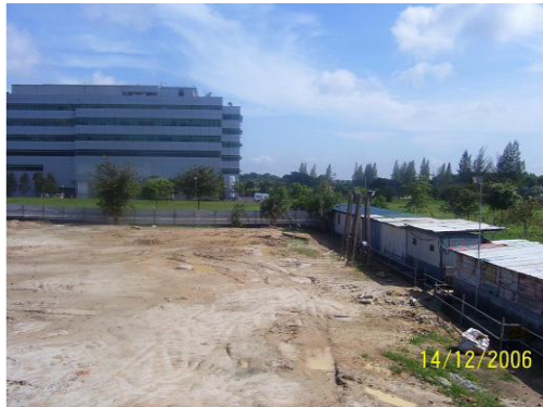
Site cleared for construction
