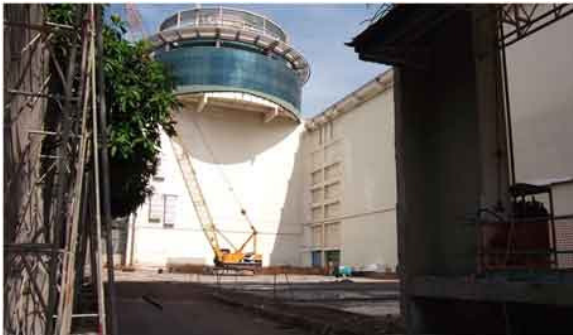
Enhancement in progress: Removal of Automated Service & Recovery System
