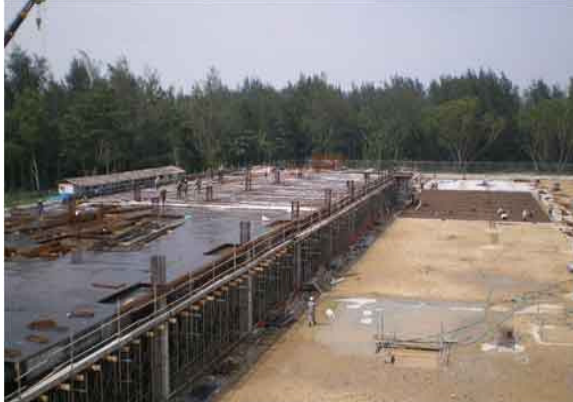
June 2011: Construction in progress
