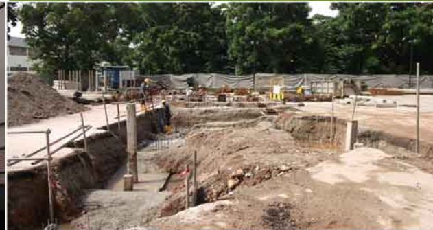
Enhancement in progress: Setting foundation for new sub-station and chiller plant
