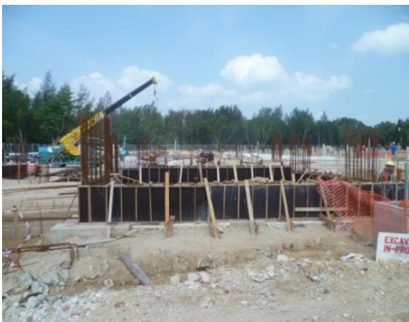
Mar 2011: Construction in progress
