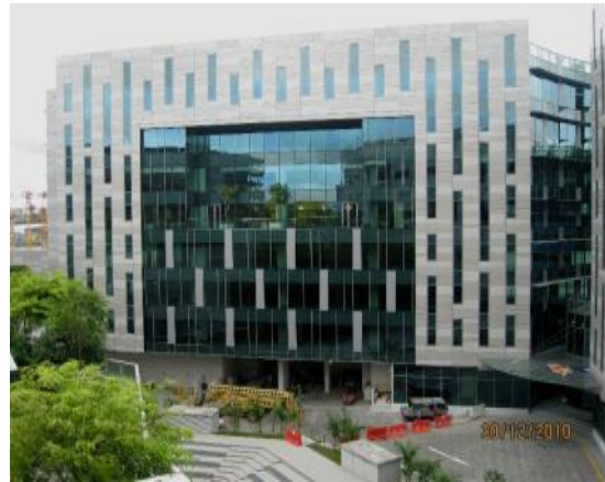
Back view of 5 Changi Business Park Crescent
