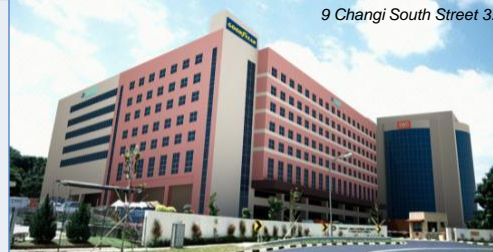
9 Changi South Street 3.
